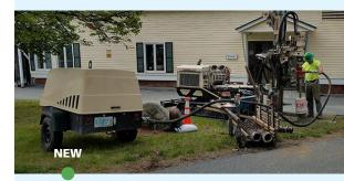
Air Hammer Unit and Compressor so rock wells can be set down to 60 feet through bedrock!
