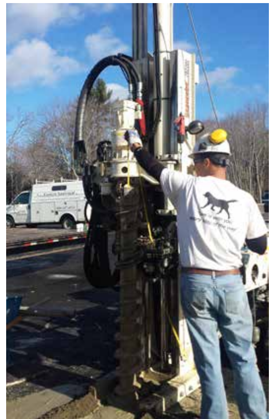
Brian installing a monitoring well
